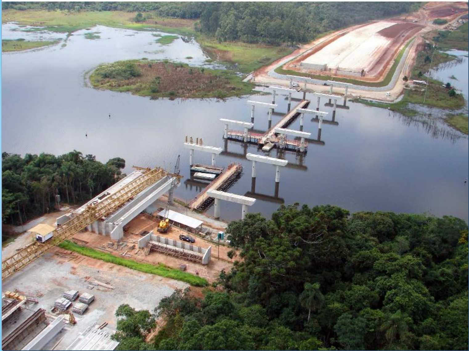
Southern Section of the Mario Covas Beltway construction details
