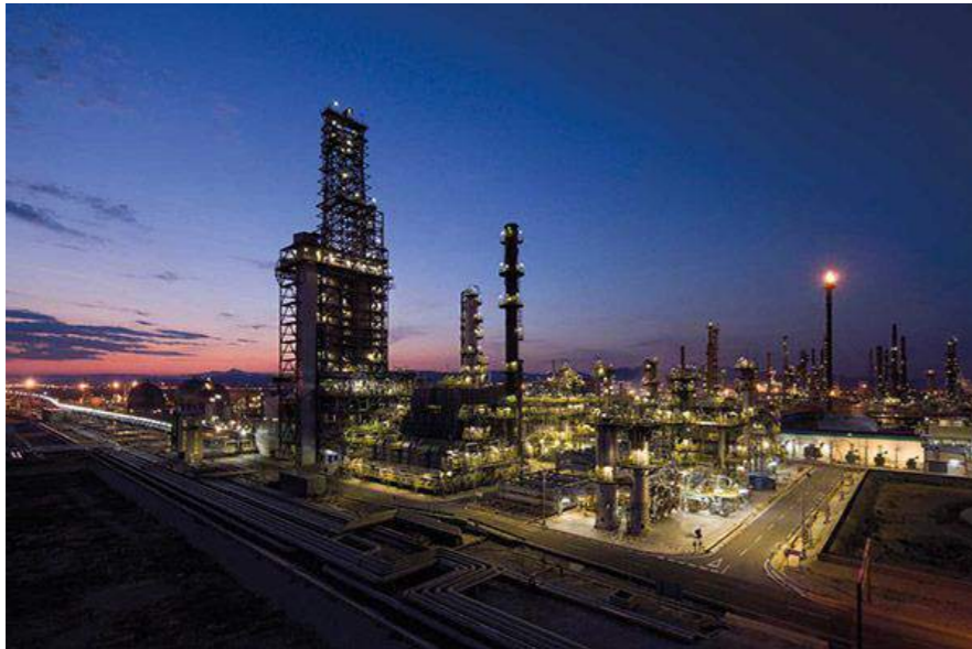
BP's Castellón oil refinery in Spain
